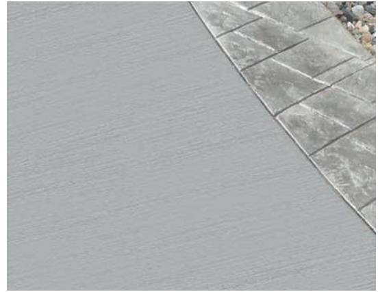
Hicrete Broom Finish Flooring
